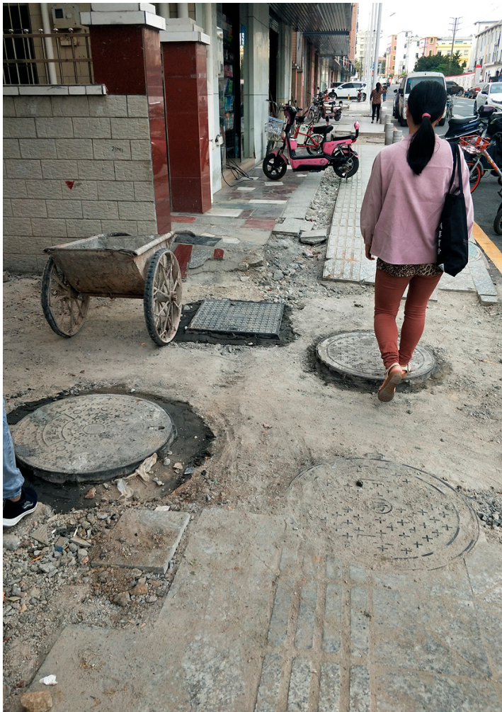
Photograph taken by one of the respondents to illustrate the continuous road construction works.
